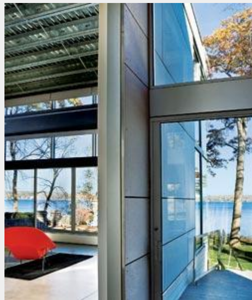
In the two-story studio, the ceiling is made of industrial joists and steel decking, the stair rails are stainless steel, and the floor is concrete.
