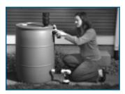
Overflow: Drill a hole near the top of the barrel to accommodate an overflow pipe that is at least 2 inches in diameter. If the overflow pipe elbow seals and seats securely, it can be threaded directly into the barrel opening. If not, it should be secured with washers on both sides of the barrel and a nut on the inside. Use Teflon tape around the threads and a bead of silicon caulking around the opening to ensure a tight seal.
